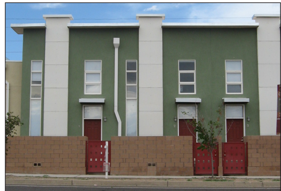
Townhouse Units - Entries face the street, garages are accessed through shared drive, and individual units are articulated
