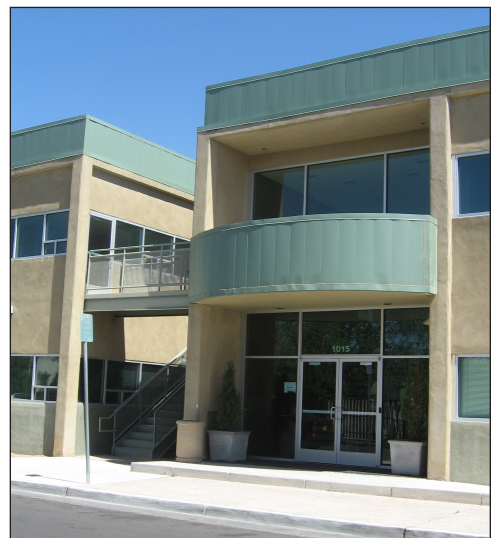
Office Building on Tijeras Ave. - entry is the predominant feature and faces sidewalk
