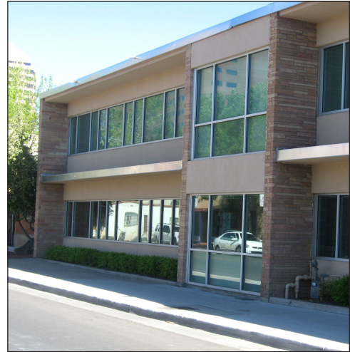
Office Building on Eighth St. - ground floor facade contains more than 50% of its surface in windows and 30% of the second story
